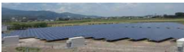
Photovoltaic Power Generation Plant (NS Saga)
