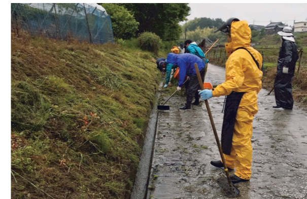
Canal Cleaning (Research Center; May 2020)
