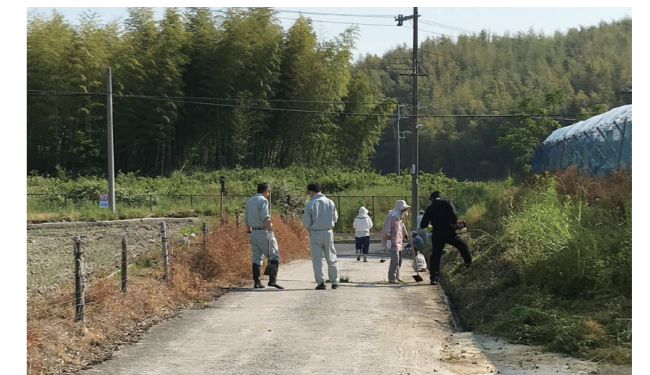
Canal cleaning (Research Center: May 26, 2019)
