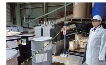
Site inspection (Nichino Service Saga - March 19, 2018)
