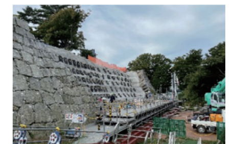
Restoration construction site
